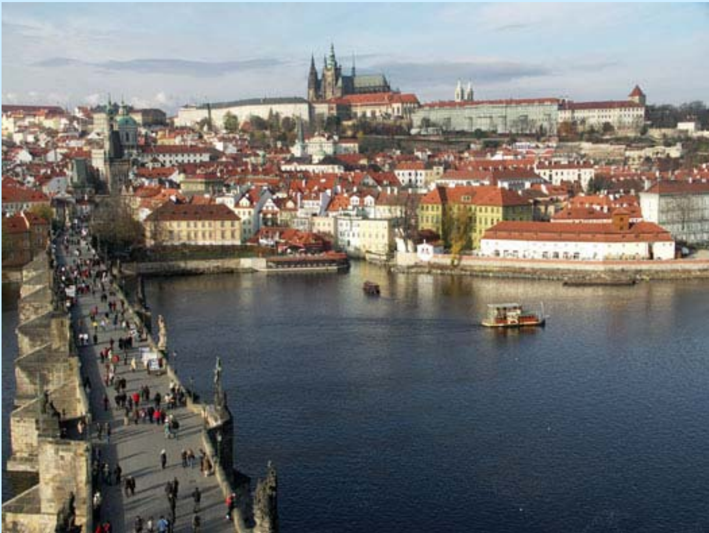
Charles Bridge – founded 1357
